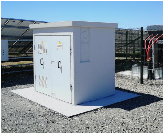
Photo 2-12: Typical cabin indoor switchgear used in the 'outdoor solution' (as per Supporting Infrastructure Option A)
