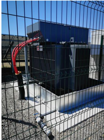
Photo 2-10: Typical outdoor transformer
