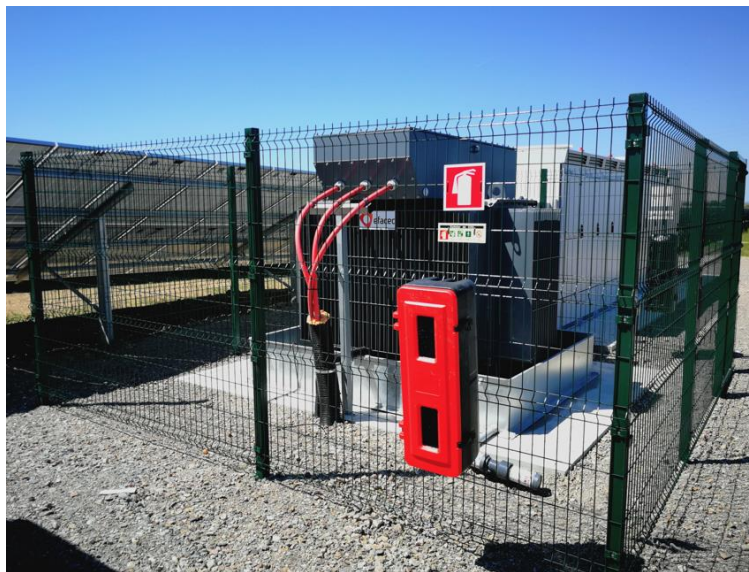
Photo 2-15: Typical transformer compound fencing
